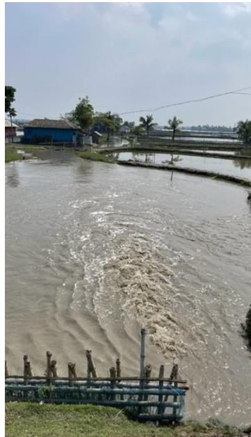
Figure 1. Salt water entering the shrimp area through the switch gate.
